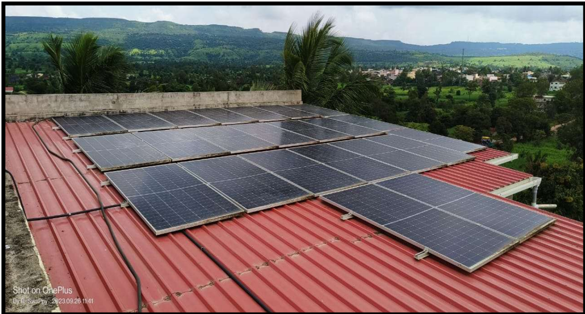
Solar Panels installation in college building
