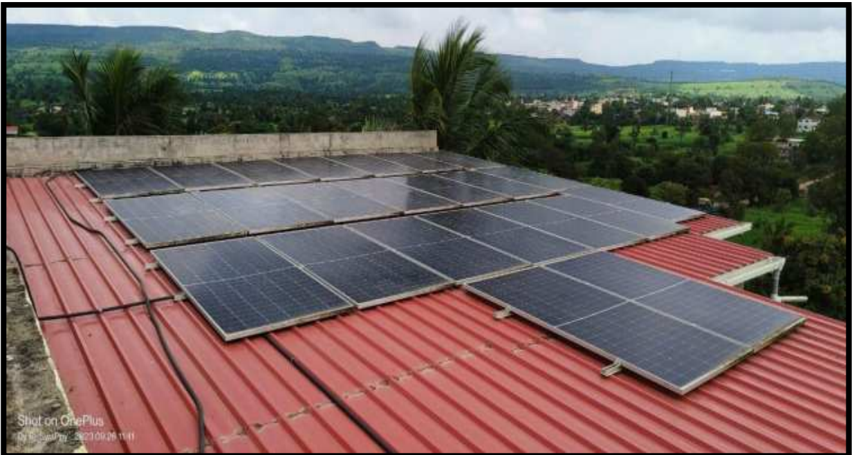
Solar Panels installation in college building
